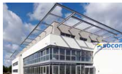
Socomec Green Building.
