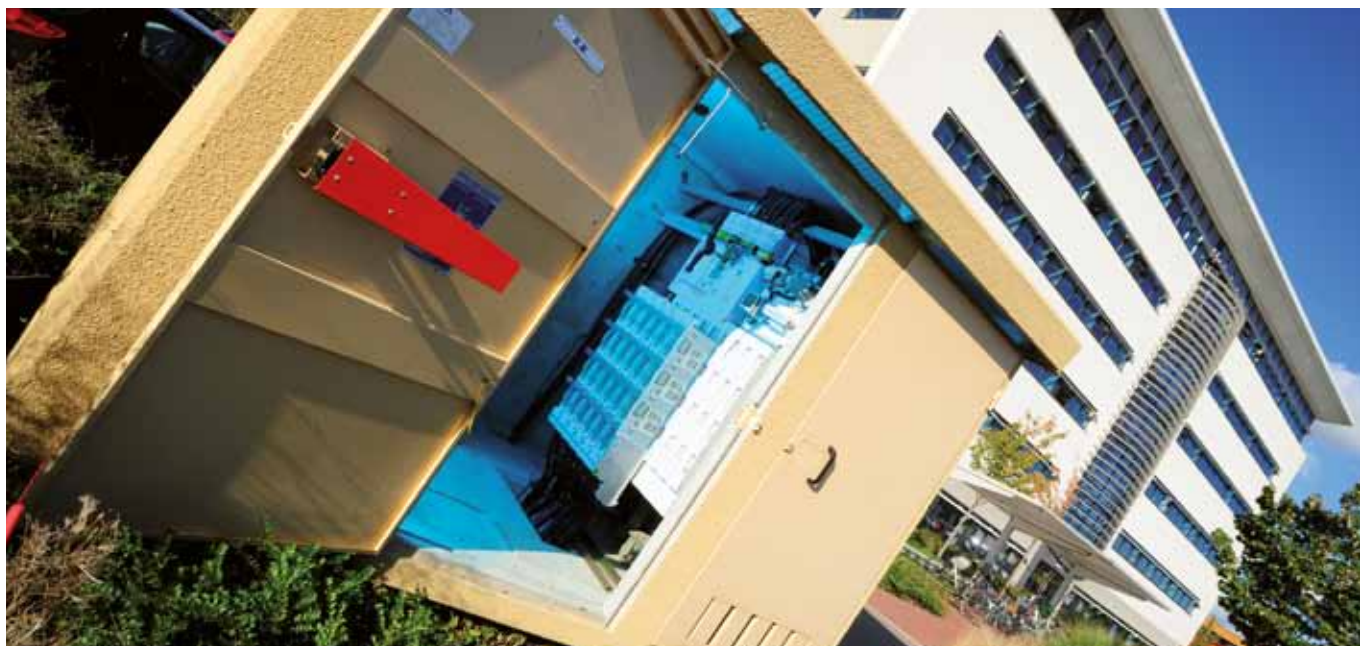
MV/LV public distribution substation with SOCOMEC TIPI feeder pillar
