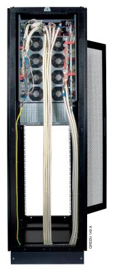
Rear view (before adding rear protective cover). Flexible cabling management for easy connections and tidier cabling.
