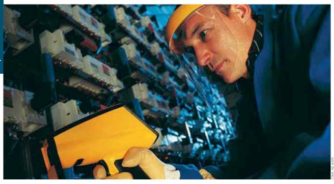
Socomec's thermal imaging service involves checking the components of your electrical installation using special infrared equipment, to ensure a high resolution analysis for predictive maintenance.
