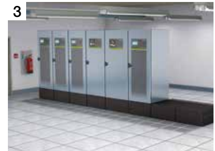
3 30 minutes later: 800 kW, online double conversion mode
